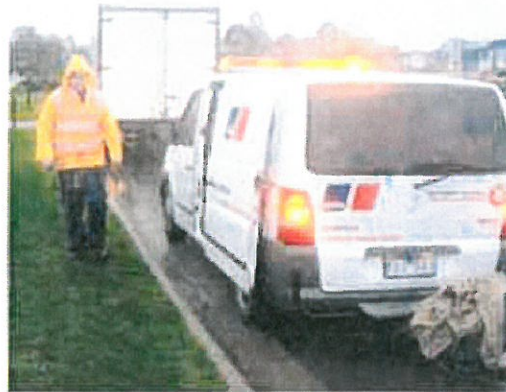
Low risk example. High visibility vests and warning lights.
