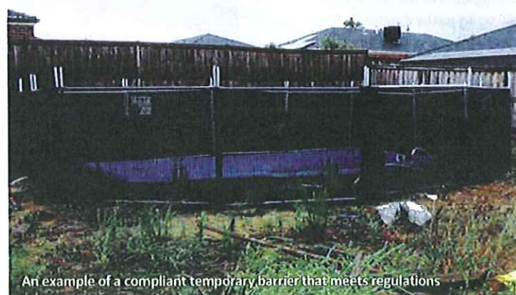
If a temporary fence isn't installed, a building or emergency order can be issued by the RBS.
