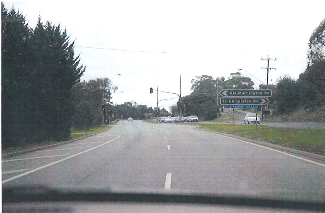
Fig 5. Image looking north on Nepean Highway, Mount Eliza, 119 metres south of the impact location at 114 km/h (4.5 seconds before impact)
